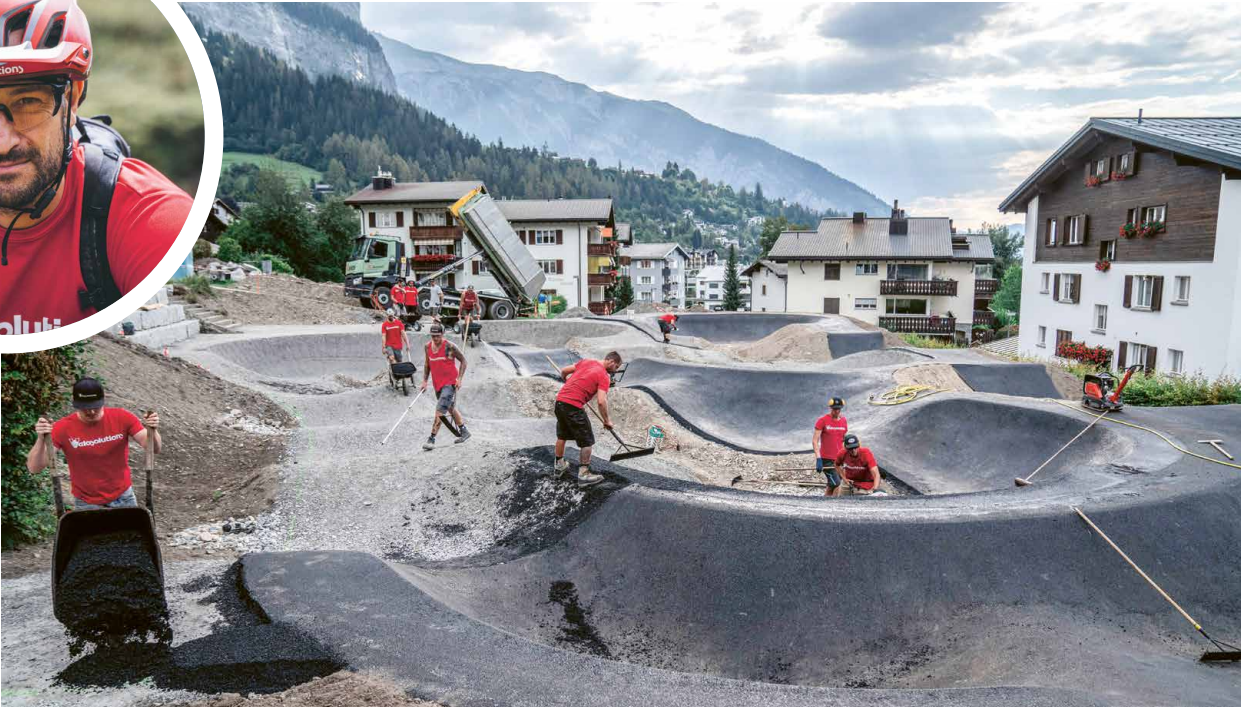
Der Pump Track in Flims während des Baus The pump track in Flims during construction
